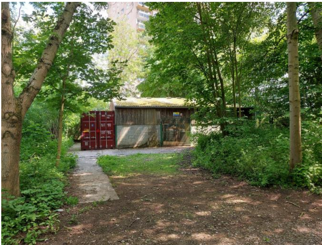
View of the container from the public footpath to the west
